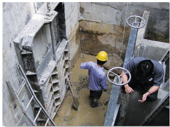
Penstock in Pumping Station, Sg. Buloh, Malaysia
